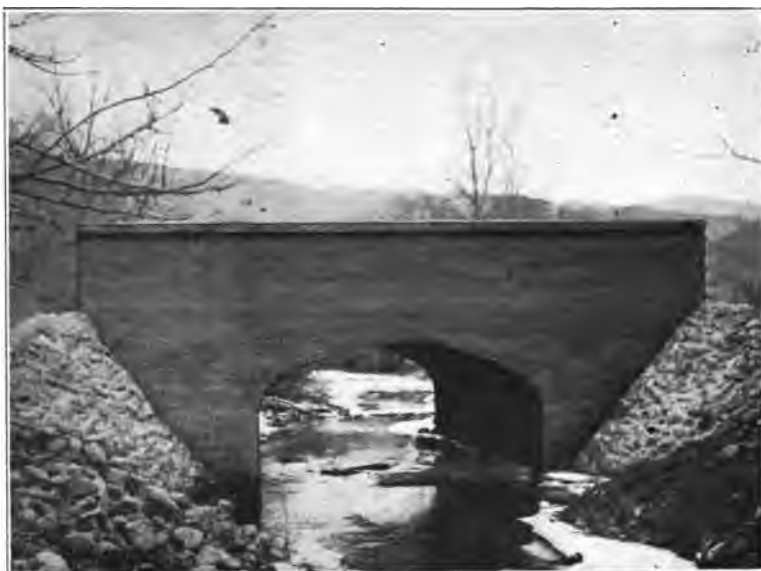
REINFORCED CONCRETE BRIDGE OVER BULLION CREEK AT MARYSVALE, PIUTE COUNTY.
